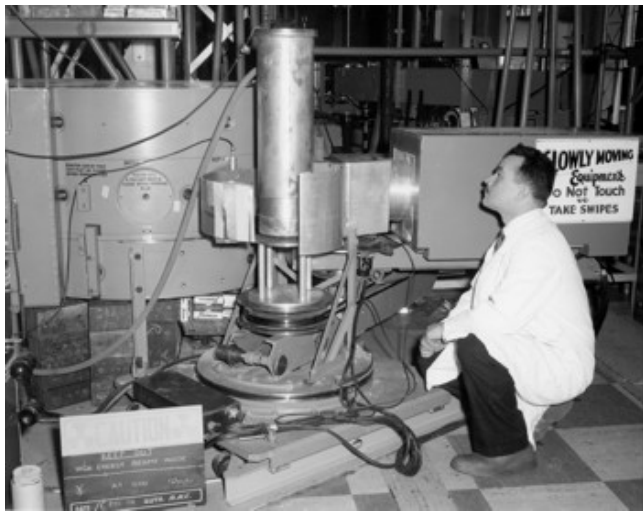
Brockhouse's first 3 axis spectrometer at NRU reactor in 1959
